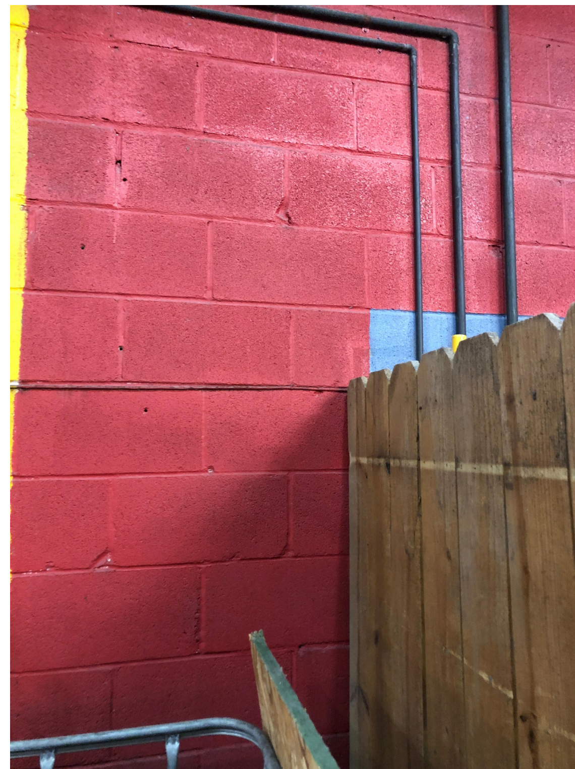
LOCATION RED PAINTED CONCRETE BLOCK REFERENCE
